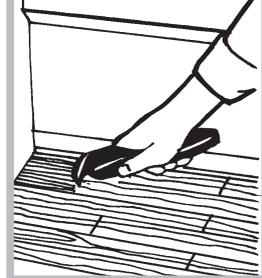
When the first rough sanding has been completed, use a broom and vacuum to clean up as much of the sanding dust as possible. Any dust left will clog the next grade of paper as you work and any grit may scratch the floor surface. It is a good idea to wear soft cotton socks on your feet as you sweep so there is no chance of grinding any of the dust into the floor with shoes.
